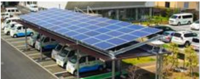
Tokyo Metropolitan Government Model Project to Promote the Adoption of Solar Carports, Hachioji Water Supply Office (Cool Net Tokyo seminar materials)
