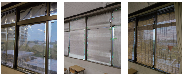
From left to right: Shading film, insulation sheets, and bamboo blinds on windows
